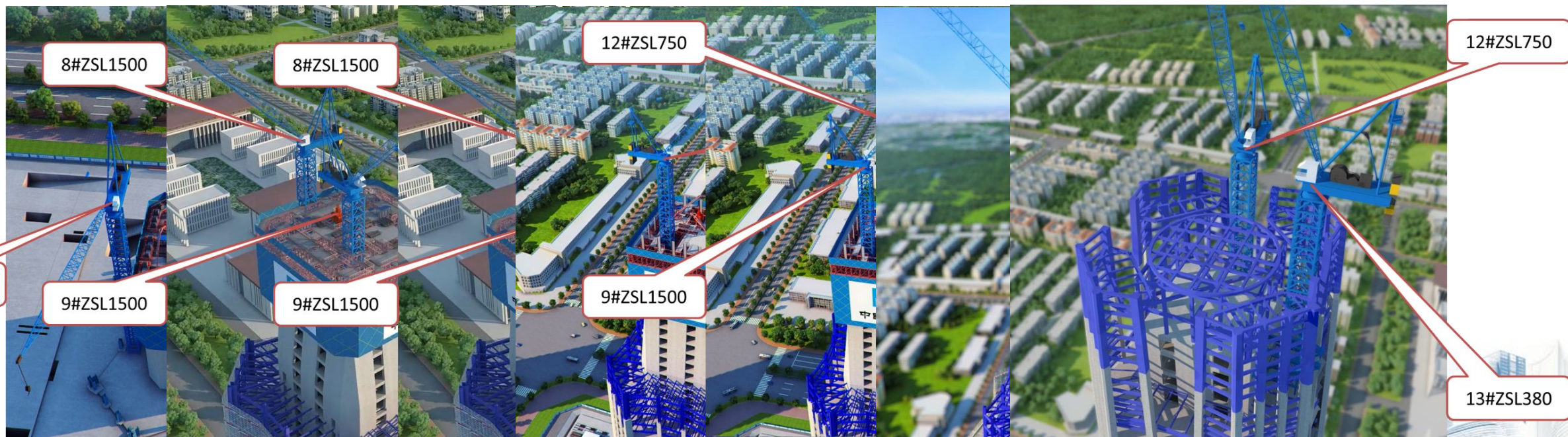
B4~4层动臂塔吊布置 7~47层塔吊布置
