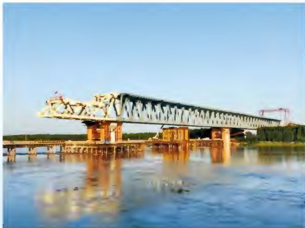
钢桁梁顶推
