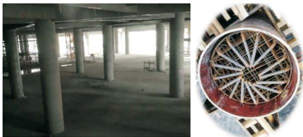
图7  $\phi 900$ 以上大截面圆柱439个
