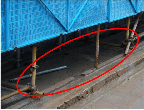
A close-up photograph of the scaffolding base. A red oval highlights the missing扫地杆 (sweeping rod) at the base of a vertical pole. |
