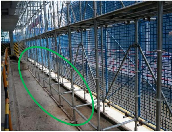
A photograph of a scaffolding structure with a blue safety net. A green oval highlights the complete扫地杆 (sweeping rod) at the base of the vertical poles. |
